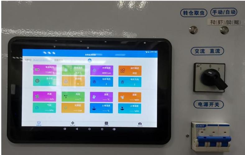
Ensure power is supplied, open the cabinet door of the measuring and reporting light through the controller panel inside the cabinet and follow the steps to check the operation of the monitor.
